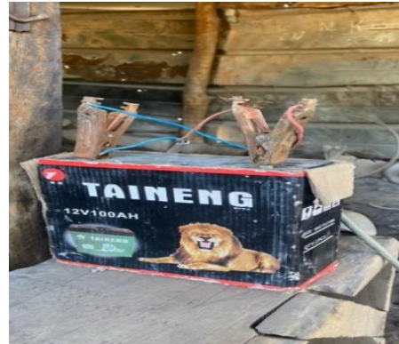
Figure 4. Engine power battery
